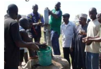
Fig. 18 Pump being tested by a WASH Officer.
