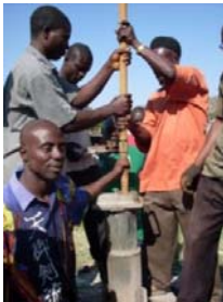
Fig. 13 Riser pipes removal
