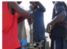
Fig. 17 Re assembling riser pipes.
