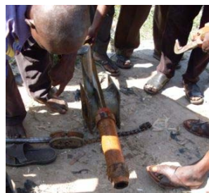
Fig.14 Pump cylinder removal
